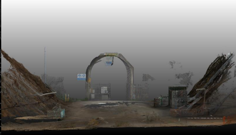
Colorized Point Cloud at Mine Portal
